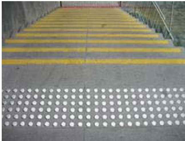
Tactile floor guidance systems in stainless steel are durable and attractive. Photos: Euro Inox, Brussels, Belgium
