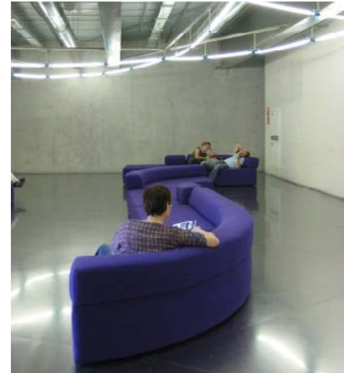
Despite its reflective character, stainless steel sheet can be made slip-resistant, as shown in the Caixa Forum exhibition hall in Madrid, Spain.
