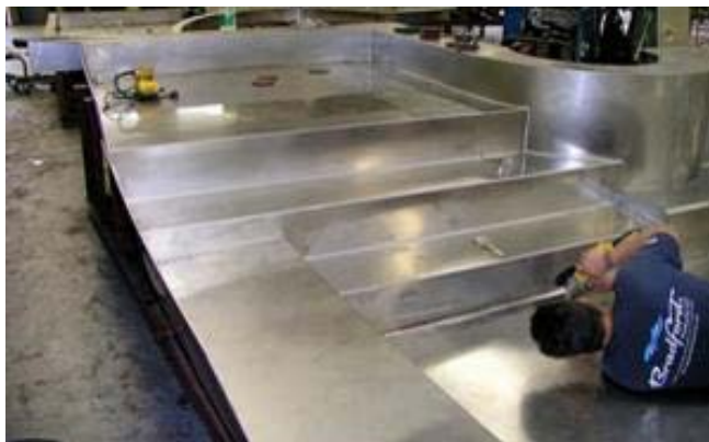
The ease of welding and polishing is a benefit when pools have to be assembled on site.
