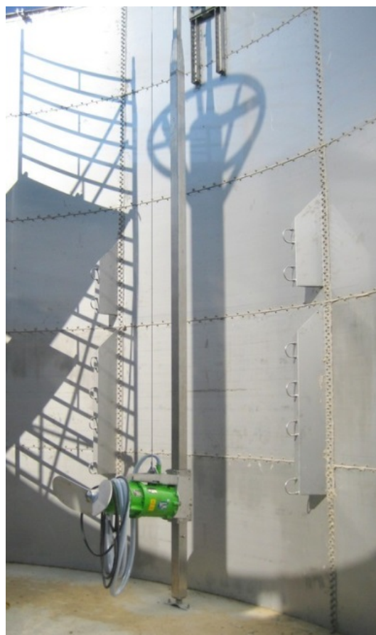
Stainless steel tanks for slurry storage and bio-gas fermentation are fast to erect and the useful life of the material is virtually unlimited. Photos: Steel Tec Farm GmbH (Germany), www.steel-tec-farm.de
