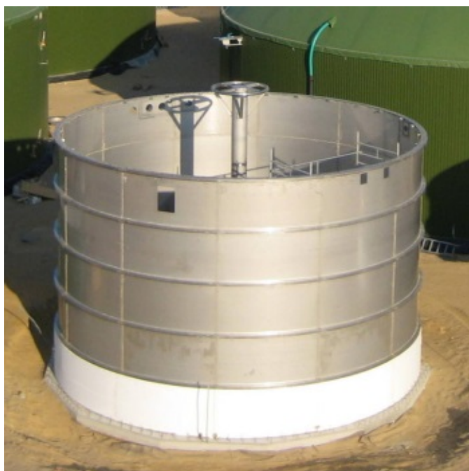
Stainless steel tanks for slurry storage and bio-gas fermentation are fast to erect and the useful life of the material is virtually unlimited. Photos: Steel Tec Farm GmbH (Germany), www.steel-tec-farm.de
