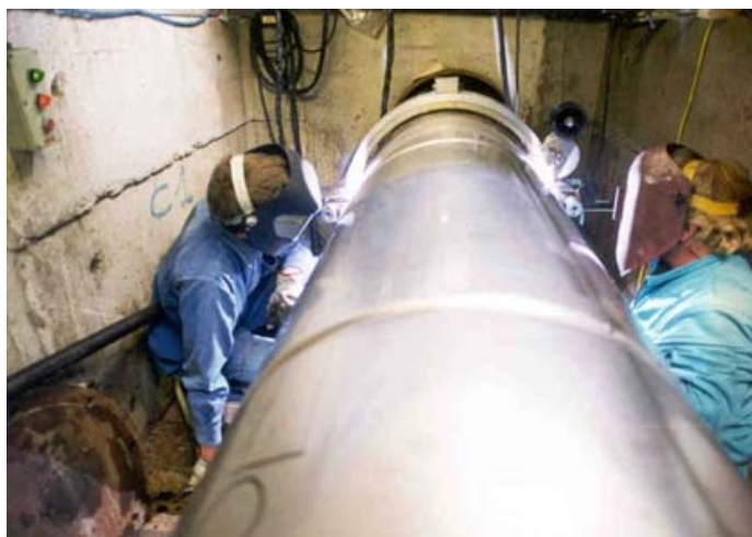
Stainless steel inserts as a repair solution for underground main supply lines.
