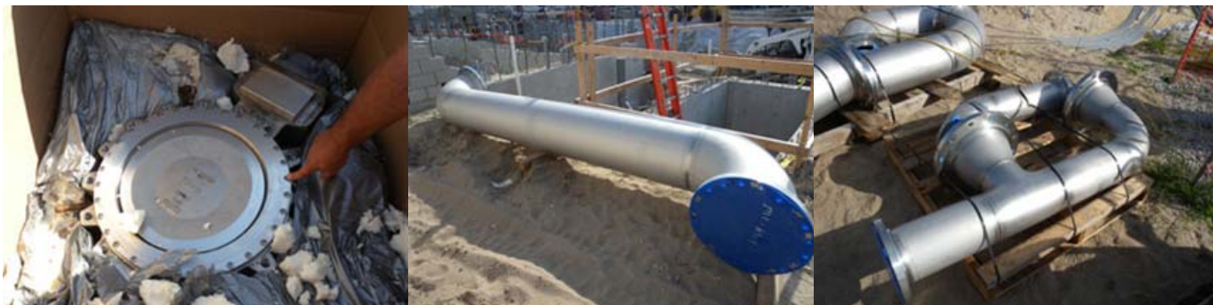
Type 316 stainless steel for the City of Lake Worth reverse osmosis water treatment plant. Source: Mock & Roos (USA), www.mockroos.com
