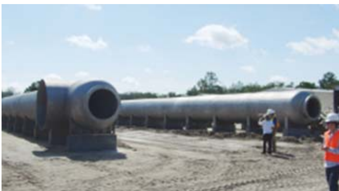
Pipework for the hydrogen sulphide removal stage of waterworks.
